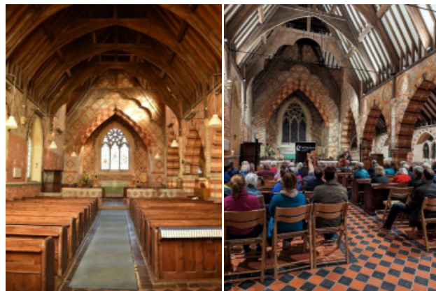
Before and after photos of the church floor
